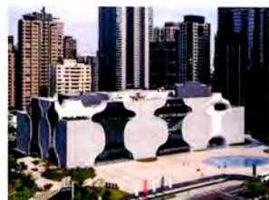
TOYO ITO National Taichung Theater Taichung, Taiwan, R.O.C.
