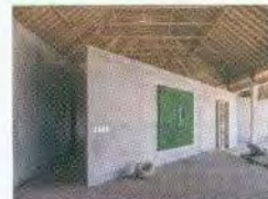
TADAO ANDO Bosco Studio & House Puerto Escondido, Oaxaca, Mexico
