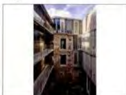
IRISARRI+PIÑERA Rehabilitation of 4 Buildings for Vigo Property Records Headquarters Vigo, Spain
